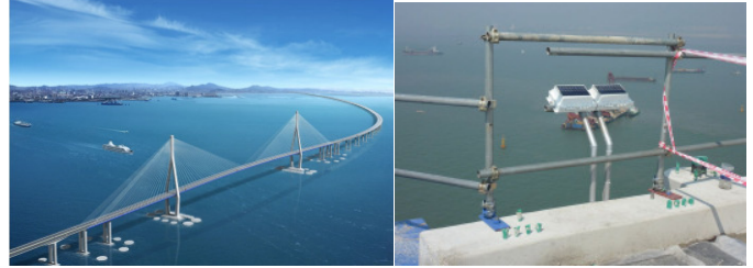
Figure 2. Incheon Grand Bridge (South Korea) with independent power supply for the monitoring system
